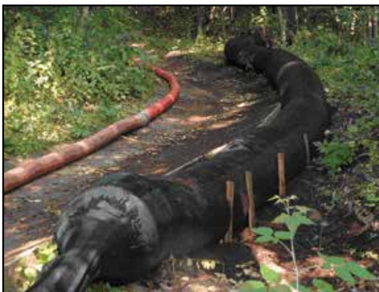
Filling Soxx for runoff diversion.
